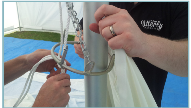
During set up. Each strap can hold over 1000kg of strength.
